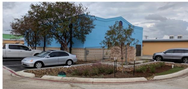
Neighborhood Place Community Center – Bioretention
