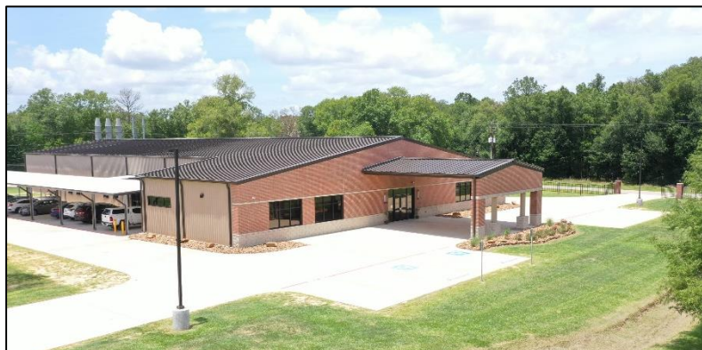
Environmental Services Division Facility
