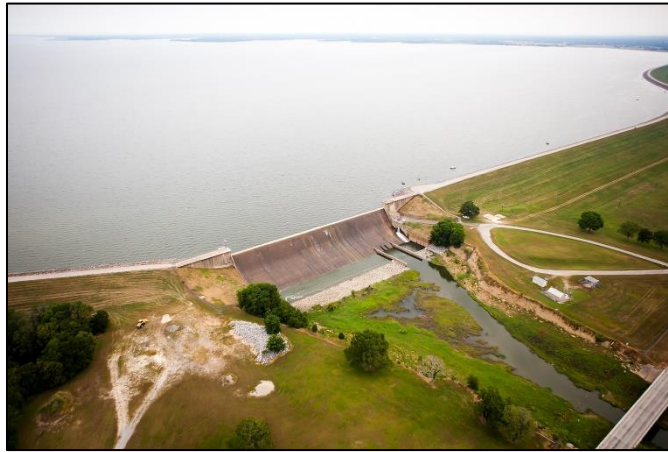
Lake Tawakoni Reservoir – Iron Bridge Dam
