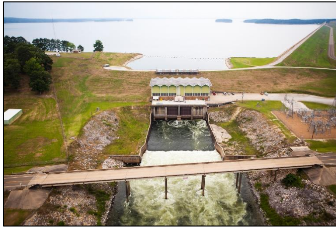
Toledo Bend Powerhouse
