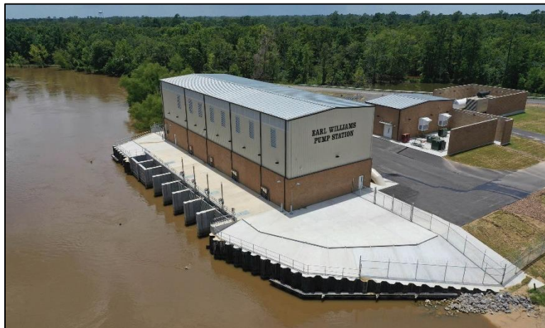
Gulf Coast Division – Earl Williams Pump Station
